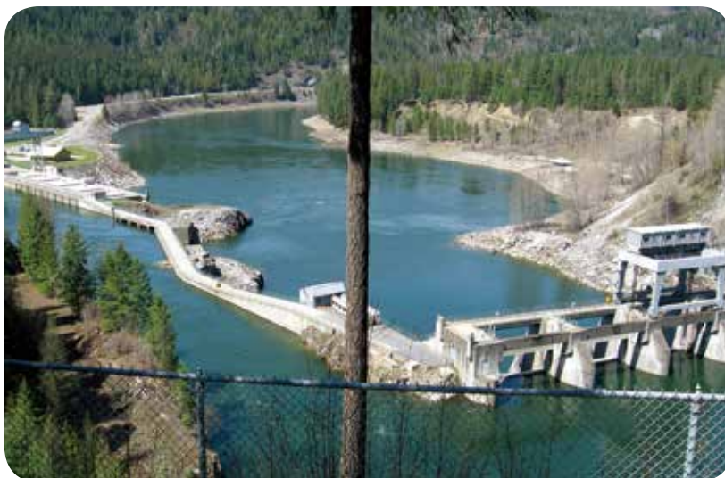
Box Canyon Dam
